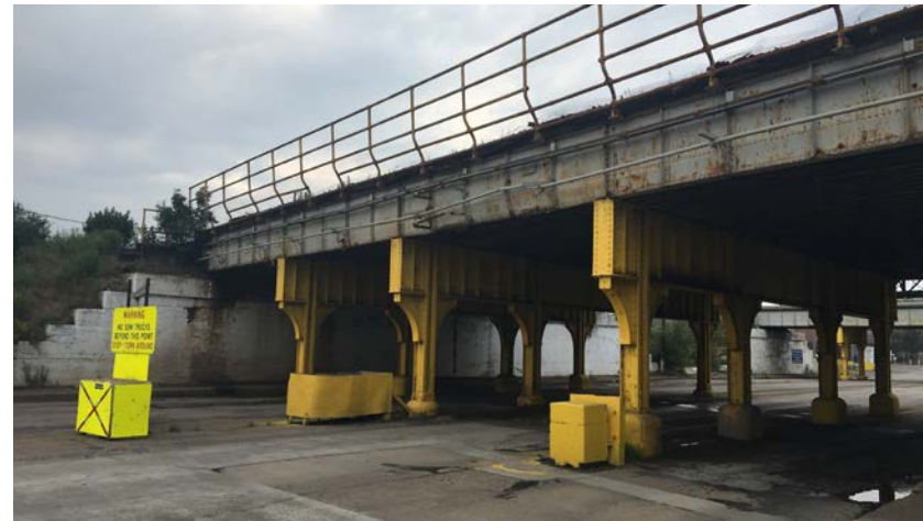
Freight rail underpass
