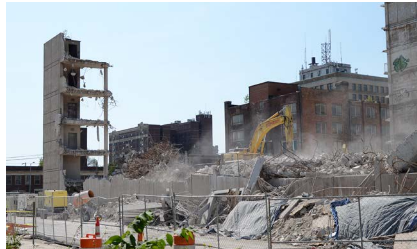
Sheraton Hotel demolition in Downtown Gary (2013)
